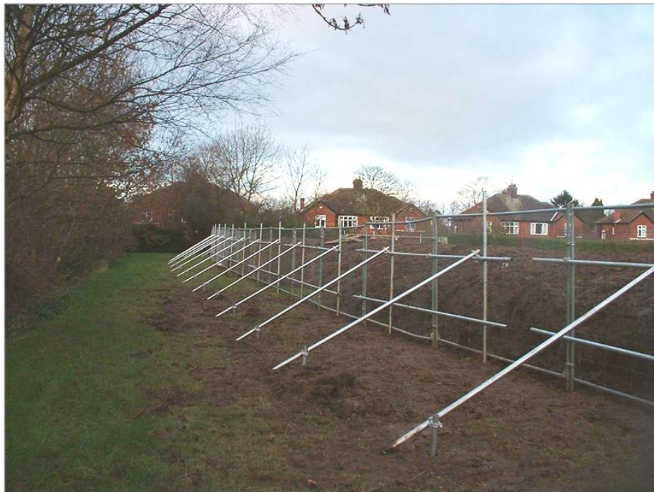
Figure 6 – Actual barrier erected on site
